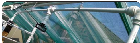
Overhead mister, starter module
